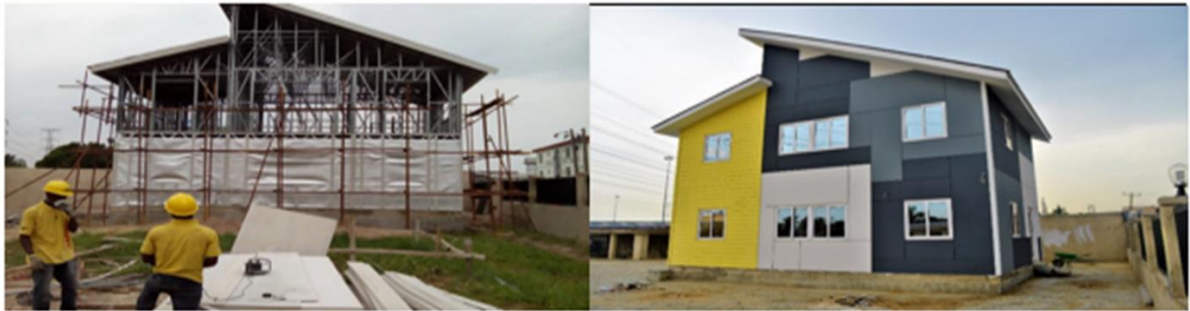
Fig. 3. DCT office building at Chevron Lekki, Lagos
