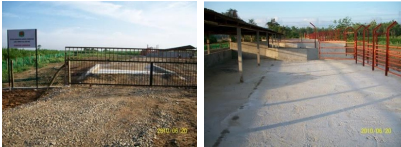
Fig. 2. KLPK Quarantine Facility [11]
