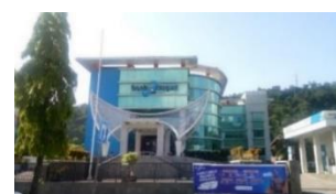
Fig. 9 Nagari Bank Branch Office
