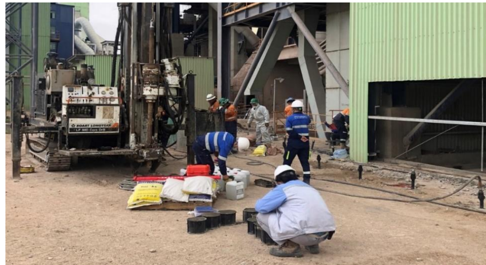
Fig.17. Photo of the process of carrying out work on cementing the soil backfilling the foundation of an industrial building
