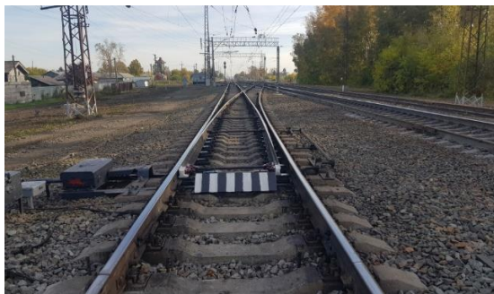
Fig. 1. A turnout of P65 type, 1/11 grade on reinforced concrete crossing sleepers
