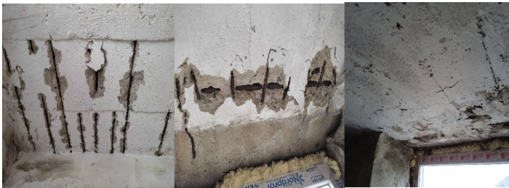
Fig. 3. General view of the ceiling condition of the silo compartment.
