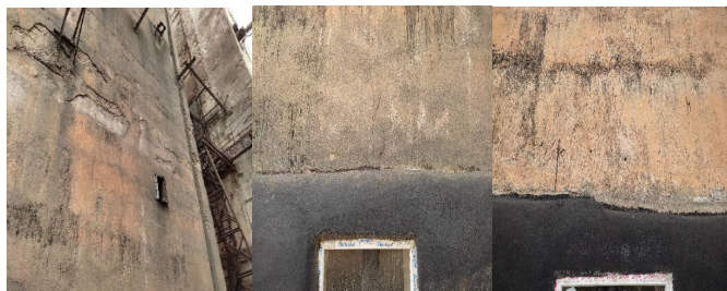
Fig. 2. General view of the condition of the load-bearing walls of the building.
