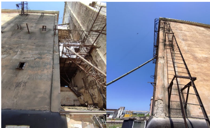
Fig. 4. General view of the condition of the columns.
