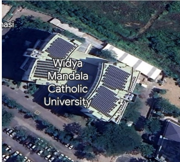
Fig. 1. Layout PV module array of 232.2 KWp rooftop and on grid Solar Power Plant located at WMSCU Pakuwon City campus.
