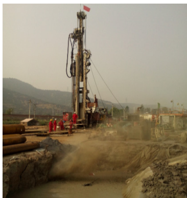
Figure 4 Effect of reverse circulation slag discharge
