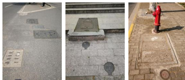
Fig. 5 Example of manhole cover (photo by author)
