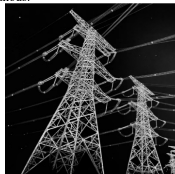
Fig. 1. Transmission tower and transmission line constructor.
