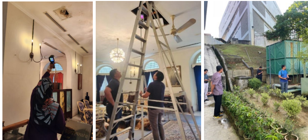
Fig. 4. The work of retrieving damage data is in progress.
