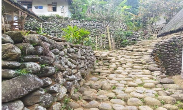
Fig. 10. Arrangement of Erosion Resisting Stone ( Entep Stone ).
