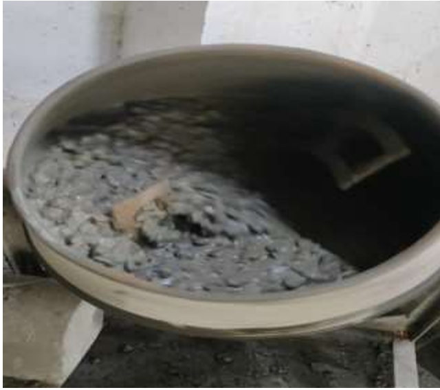
Figure 5: Mixing of Concrete
