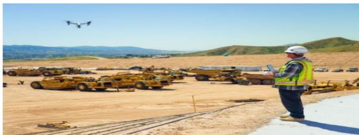
Fig.11 Scanning of the construction site https://id.foursquare.com/v/one-timedevlopment-company/5a5ccf3f42d8c2565f680676
