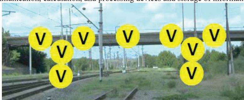
Fig. 7. The scheme of the study areas in the system of monitoring the condition of overpass structures above the railway
