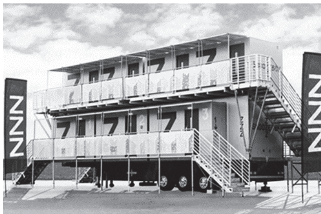
Fig. 3. Mini-hotel from containers “Snoozebox” based on a car chassis (Great Britain, 2013)
