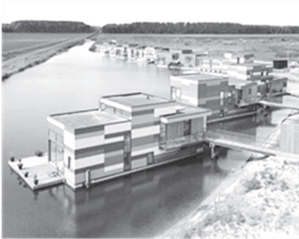
Fig. 4. Floating houses on pontoons (Amsterdam, Netherlands)
