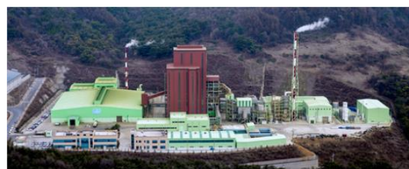
Fig. 6. Ausmelt TSL Plant operated by GRM
