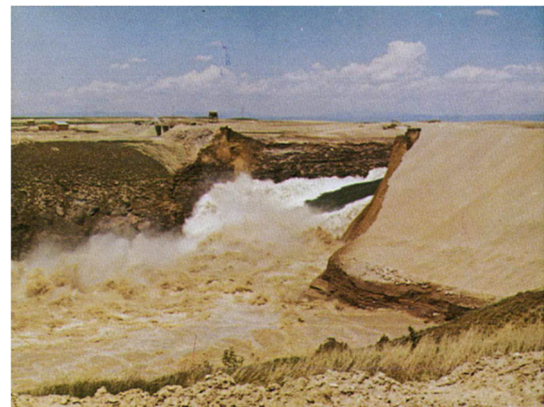
Figure 1. Teton dam was destroyed (Independent panel to review the cause of Teton dam failure 1976).
