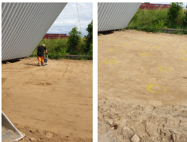
Figure 6. Compaction and preparing of the subgrade soil in the test pit.
