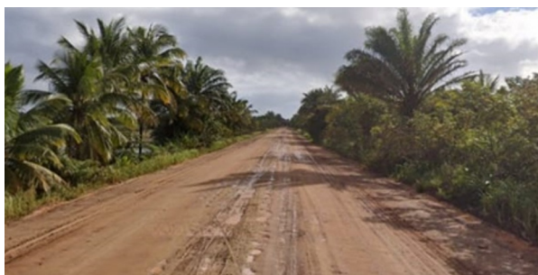
Figure 3. Frontal view of the region where the test section will be implemented on the BR-030/BA highway
