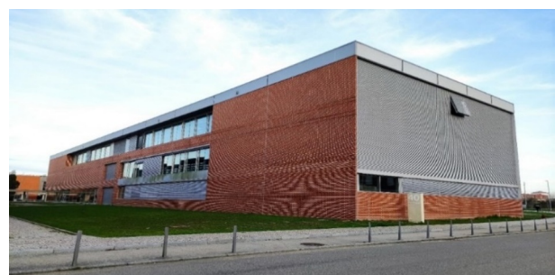
Figure 3. The building under study: south and west façade views.
