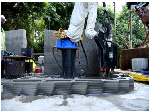
Fig. 1. 3D Printing in Progress in KESNIK Campus, India.
