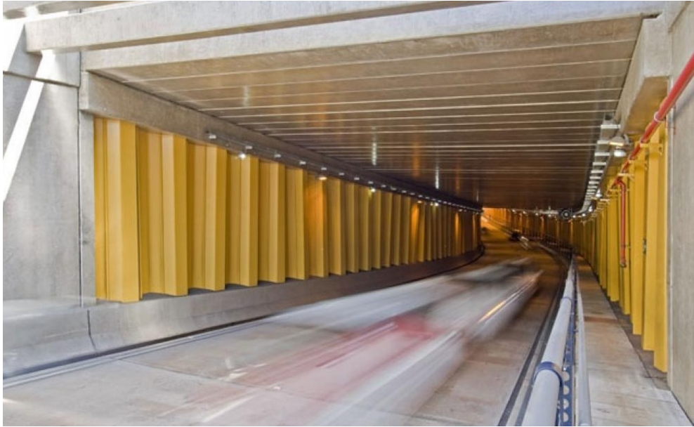
Fig. 7. Underground structure with walls - steel sheet piles in Brazil.
