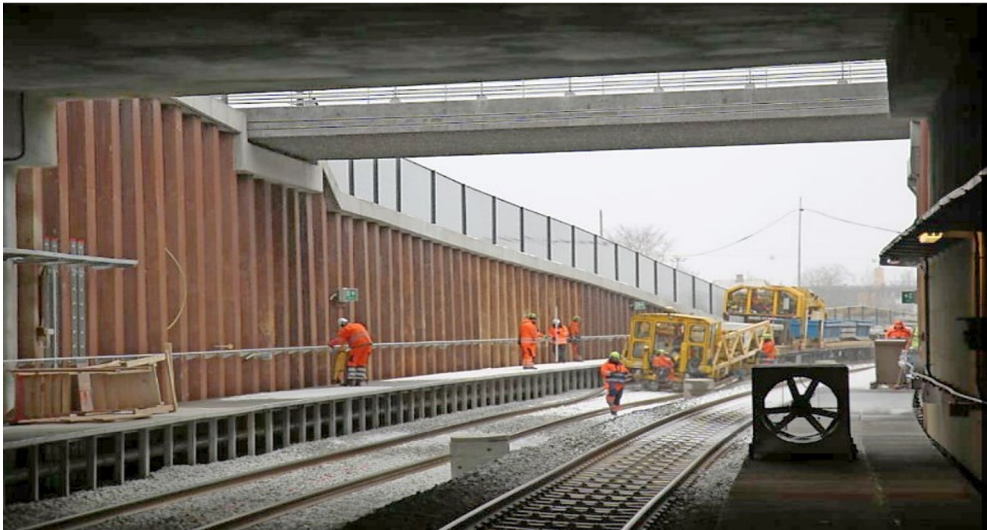
Fig. 5. Overpasses above the high-speed railway line Copenhagen-Ringsted, Denmark.
