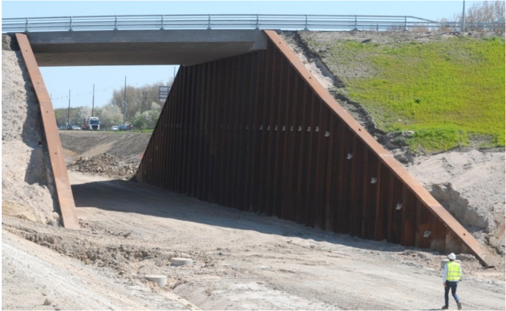
Fig. 8. Road overpass L~13m with integral abutment (Copenhagen-Ringsted railway line), Denmark.
