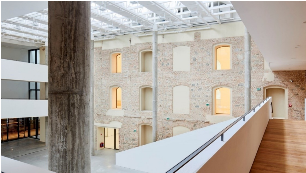
Fig. 3. View of the restored wall with new structures around it [10].
