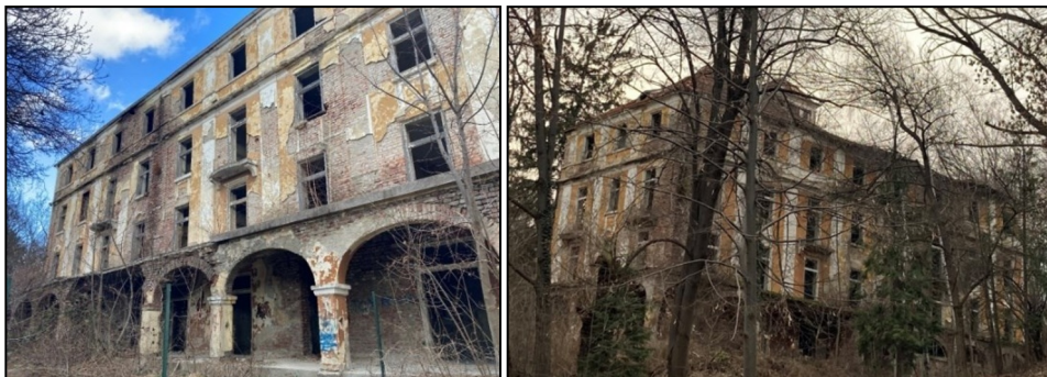
Fig. 1. General view of the building and its present condition.
