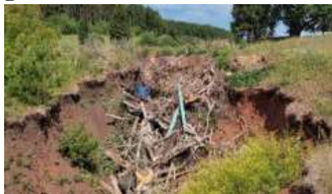
Fig. 3. Gully on the floodplain of the Varzinka River resulting from the breach of two earthen dams of the ponds: A - photo in July 2008; B - photo in July 2023
