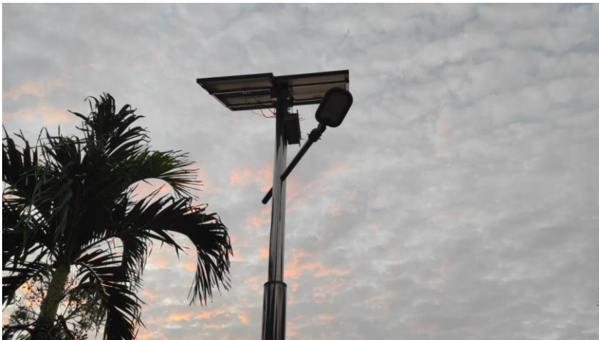
Fig. 8. The Installation Off-Grid Solar Power Plant
