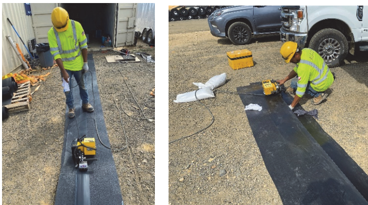
Fig. 1. Photographs of Fusion or wedge welding/seaming of HDPE geomembrane
