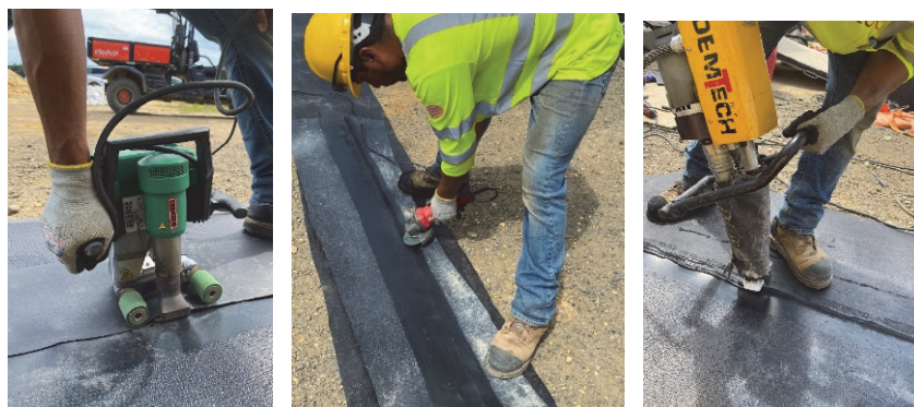
Fig. 2. Photographs of the extrusion welding/seaming of HDPE geomembrane process
