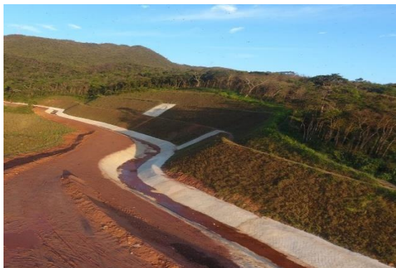
Fig. 5. Spillway Structure of a Tailings Dam, Minas Gerais.
