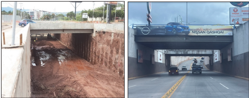
Fig. 6. Project 3 Juan Pablo II Boulevard Underpass. Before (2016) and after (August, 2023)
