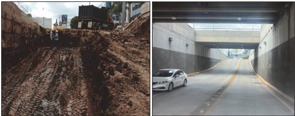
Fig. 4. Project 2 Boulevard Juan Bosco at M.D.C., Honduras. Before (2019) and after (August, 2023)
