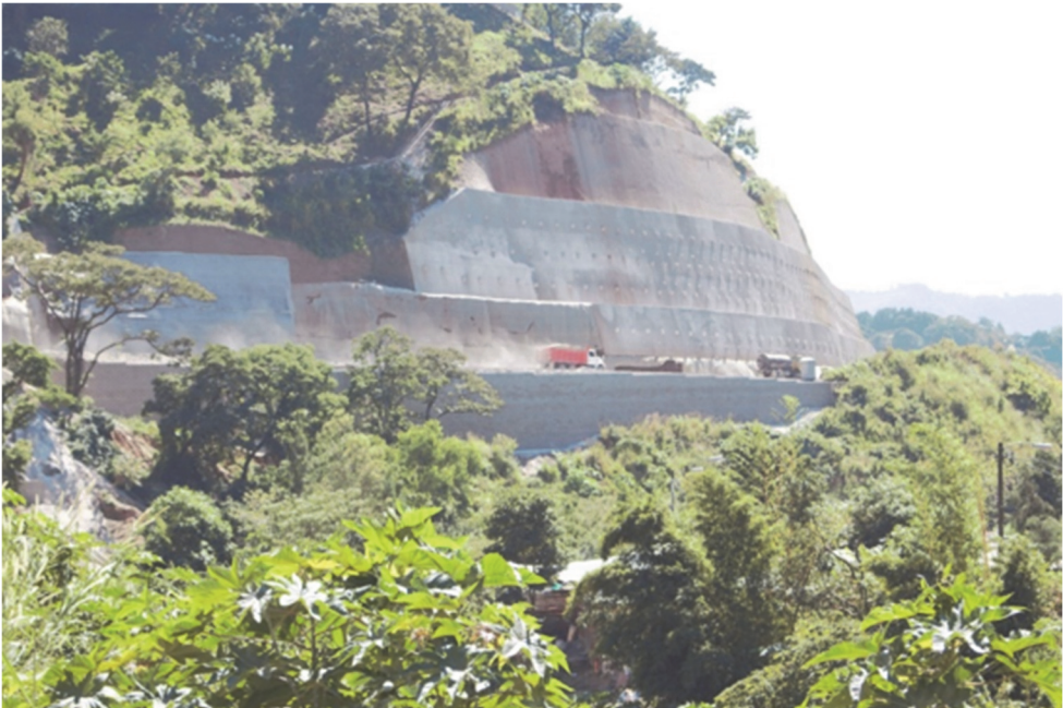
Figure 3. Panoramic of MSE wall and anchors after construction
