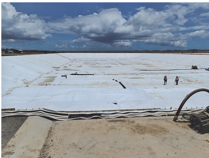
Figure 3. White HDPE installation works at Yarwun Refinery Caustic Bladder
