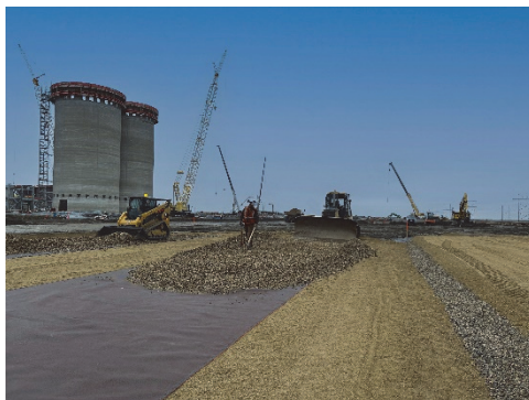
Fig. 1. Placement of high-modulus woven geosynthetic between ballast & sub-ballast
