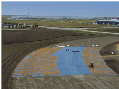
Fig. 2. Placement of MMG on subgrade of railway structure
