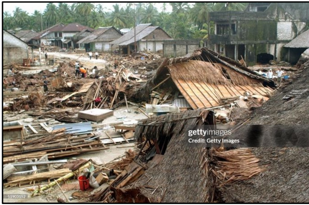
Fig. 3. Houses destroyed at Sirombu (source: getty images, 51903152, december 29, 2004)
