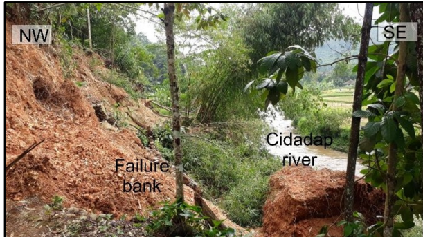
Fig. 7. Failure at Cidadap River bank
