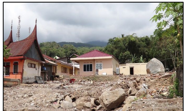
Fig. 1. The collapse of an elementary school and residential area in Nagari Koto Tuo due to flash floods following the eruption of Mount Marapi in West Sumatra.
