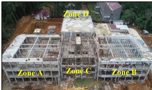
Fig. 1. The Central Laboratory Building of Universitas Andalas
