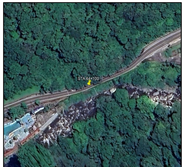
Fig. 1. Landslide location in Padang Panjang-Sicincin Road section (STA64+100) [2]
