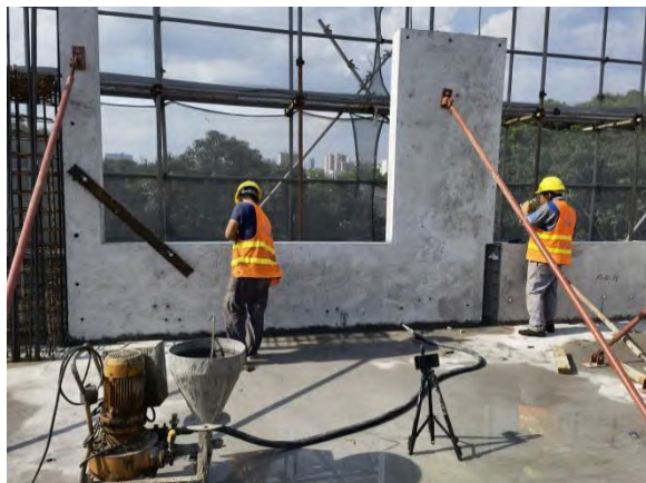
Fig. 5 Grouting method construction [13].
