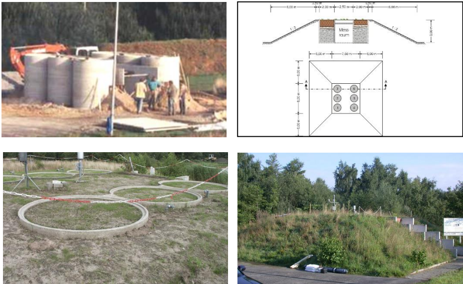
Fig. 1: Impressions from the construction of the lysimeters
