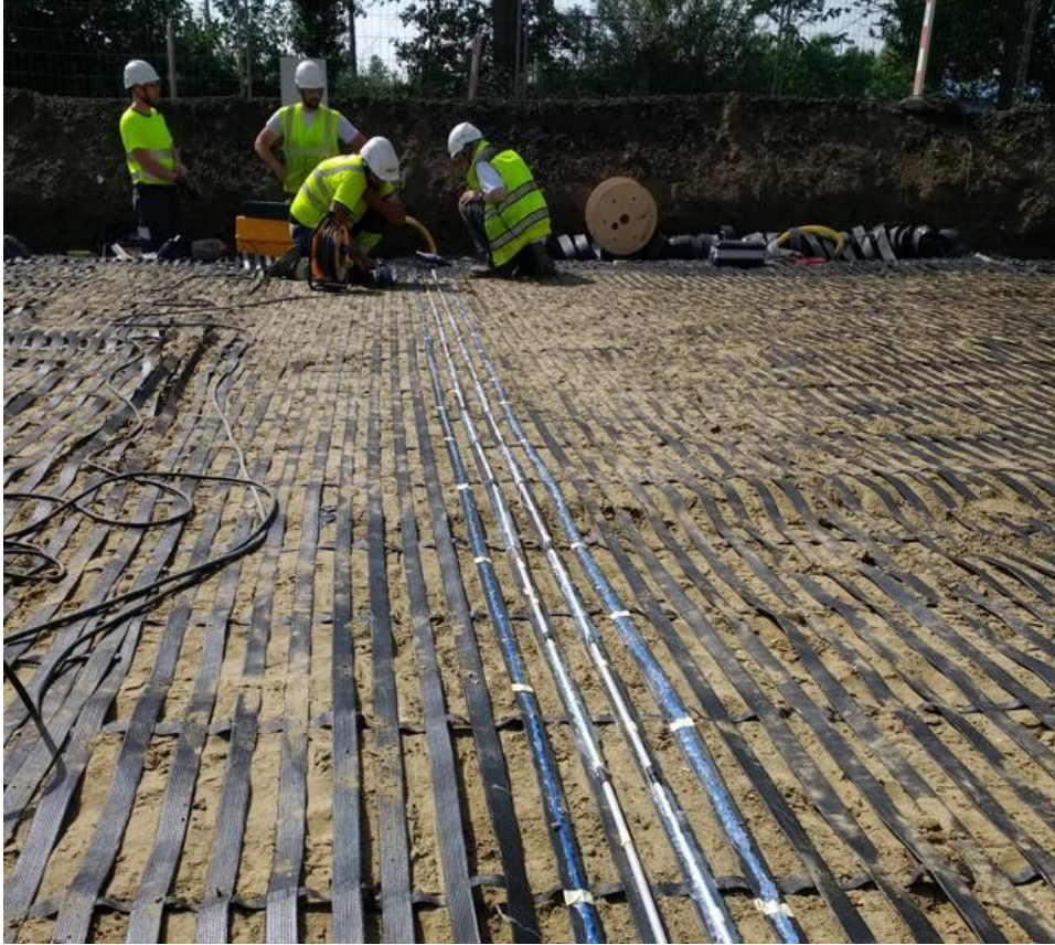
Fig. 8. Instrumentation of the first level of geogrid to be monitored
