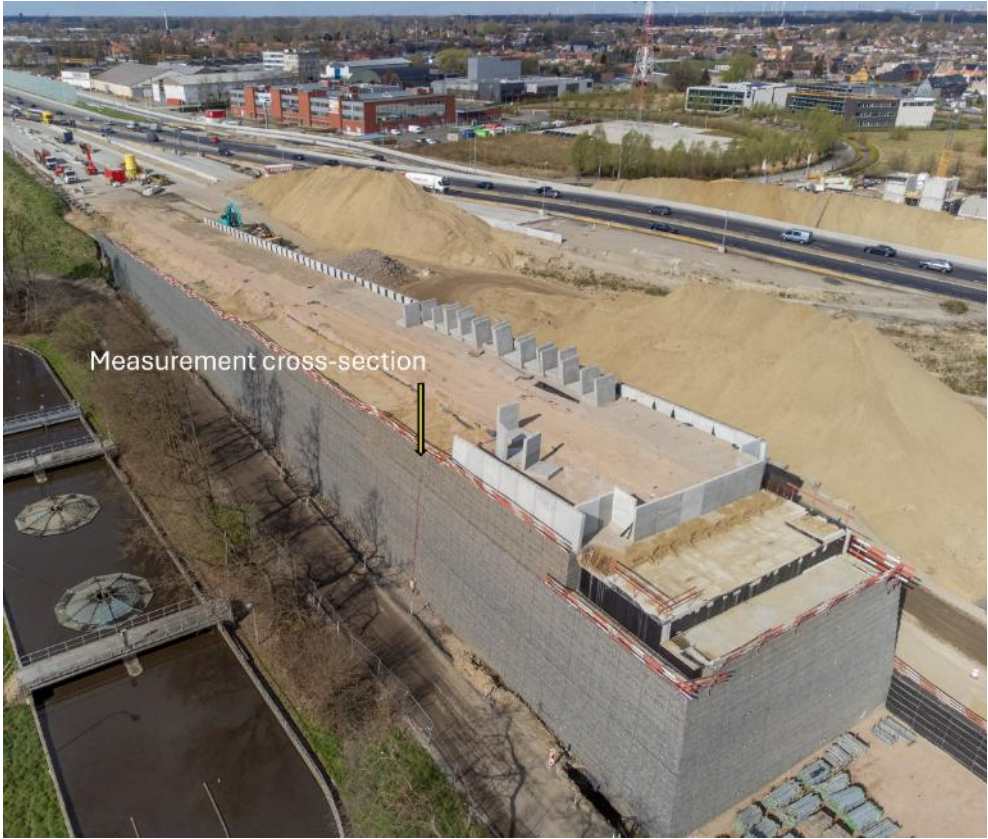
Fig. 3. Reinforced fill structure to be monitored under construction.
