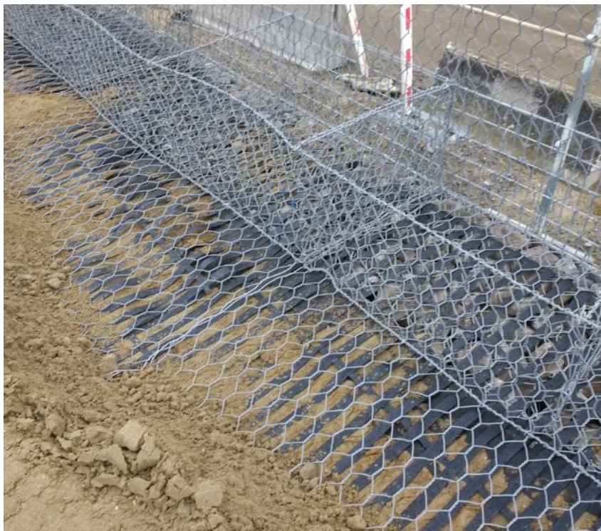
Fig. 5. Installation of the different geogrid and facing components on the field
