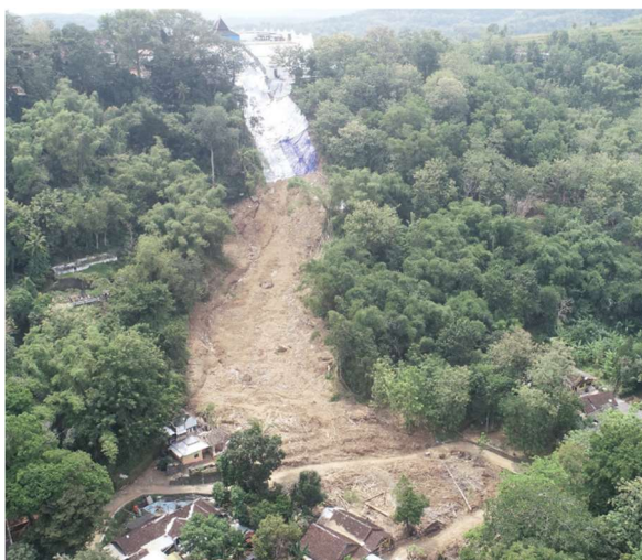
Fig. 2. Existing conditions after landslide
