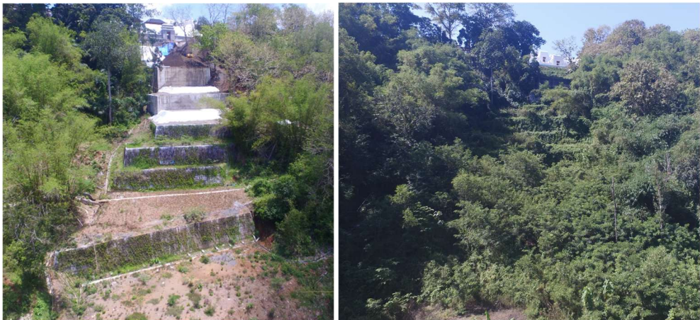
Fig. 10. Slope reinforcement several months after construction and current slope conditions
