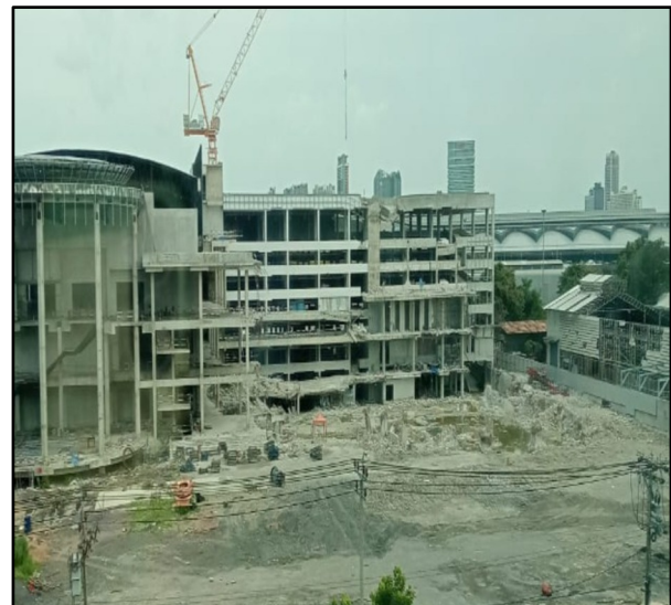
Fig. 3. The rest of the building ruins are still in the construction work stage.
