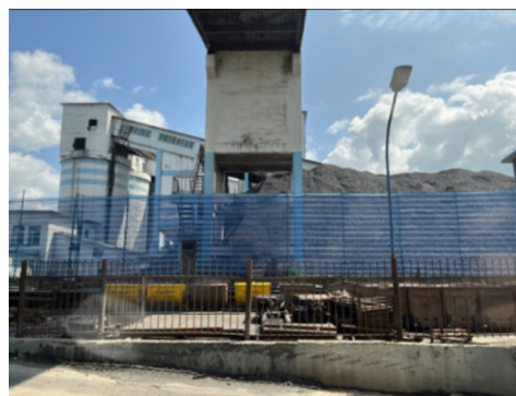
Figure 8. Opened coal yard with windbreak dust suppression nets
