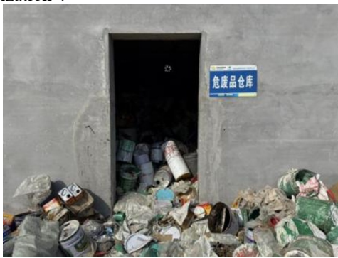
Figure 10. Waste paint buckets were disorderly stacked in warehouses without doors and impermeable floor
