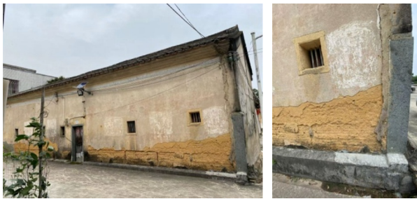
Fig. 3. The Erosion and Protection Quo of the Hakka Rammed House (Author Source)
