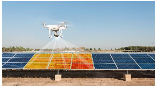
Fig. 9. Thermal inspection of a photovoltaic plant.
