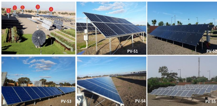
Fig. 6. Green Energy Park platform in Morocco with different technologies of photovoltaic modules [9].
