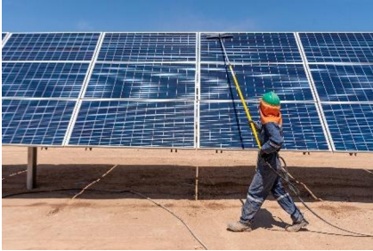
Fig. 7. Manual cleaning of photovoltaic modules.
