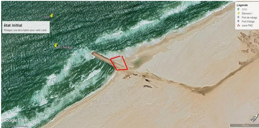
Figure 8: Start of construction works at N'diogo port (image 2018-04).
