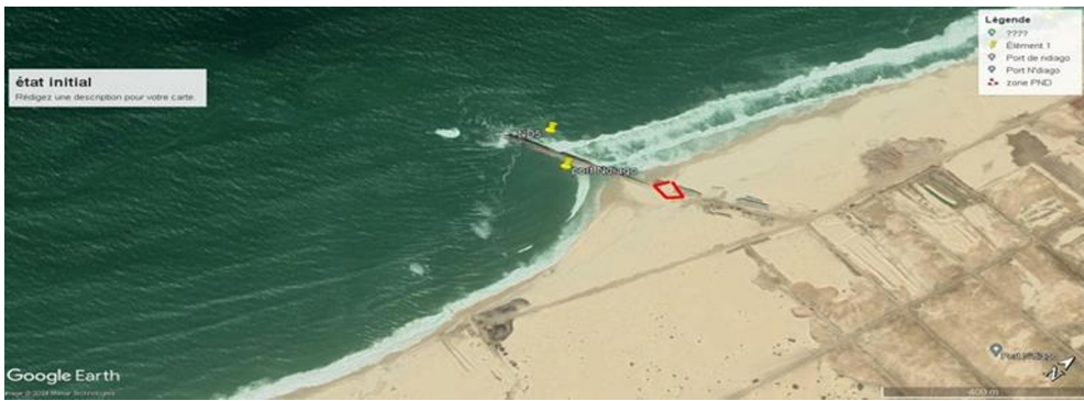
Figure 9: Seven months after the construction of the breakwater at N'diogo port (image 2018-11).
