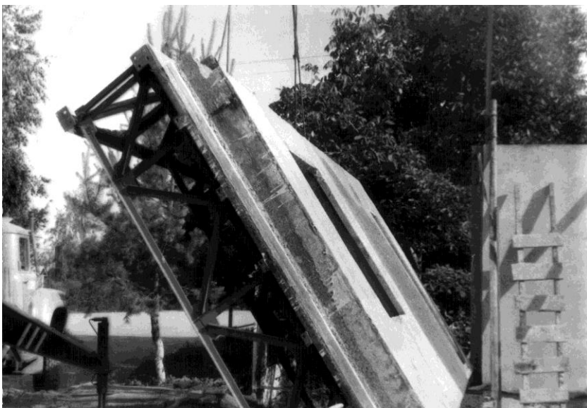
Fig. 4. Lifting a three-layer wall structure using a truck crane.
