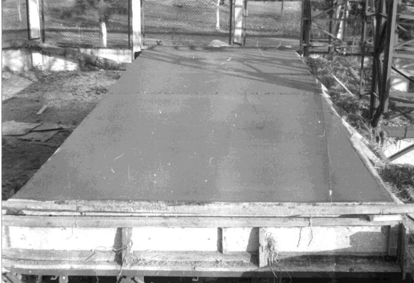
Fig. 3. Curing the structure until the concrete reaches its installation strength.
