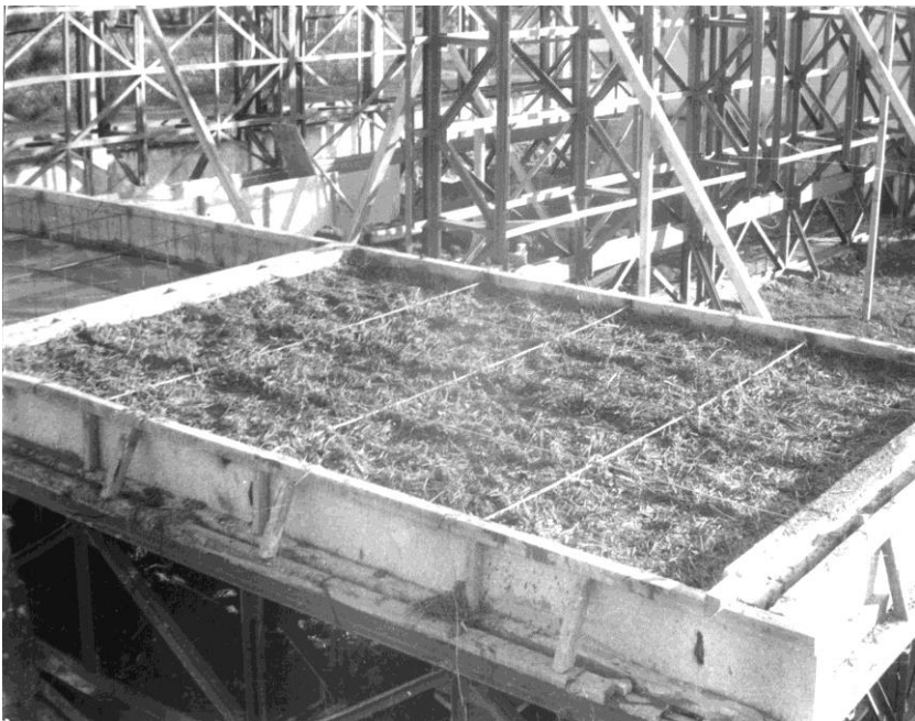
Fig. 2. Wood-cement mixture placed in the formwork.
