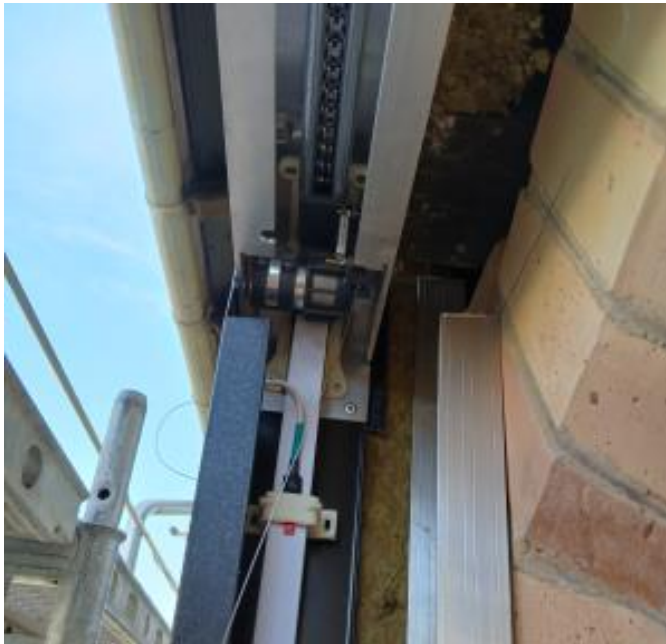
Fig. 8. IWS frame and electric engine on the corner and the moving mechanism on the top.
