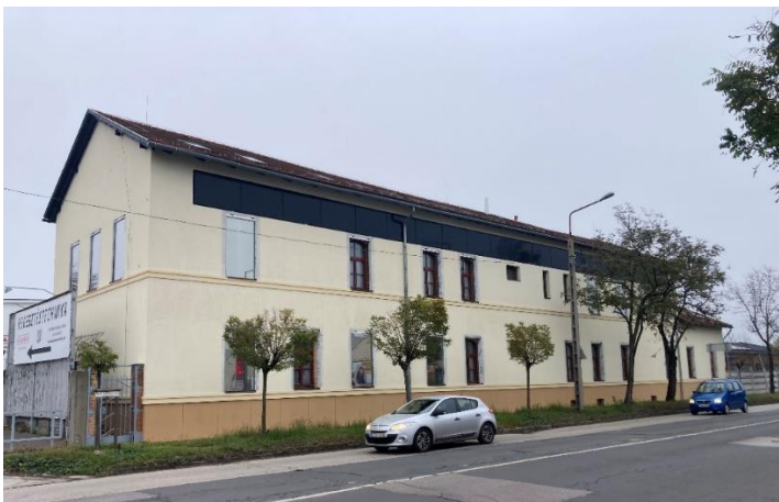
Fig. 10. The Hungarian demo building after renovation.
