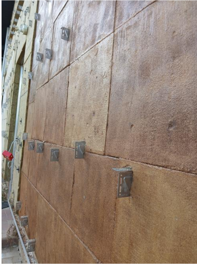
Fig. 7. Experimental fixing of Activated Cellulose to the wall of the demo site.
