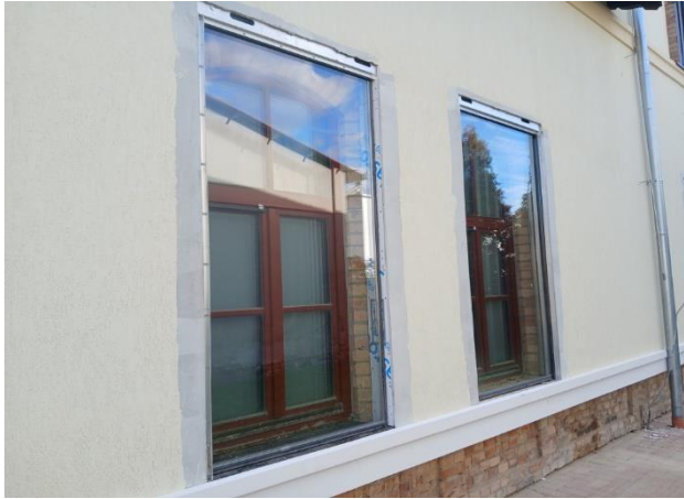
Fig. 9. Installed IWS in front of the existing window.
