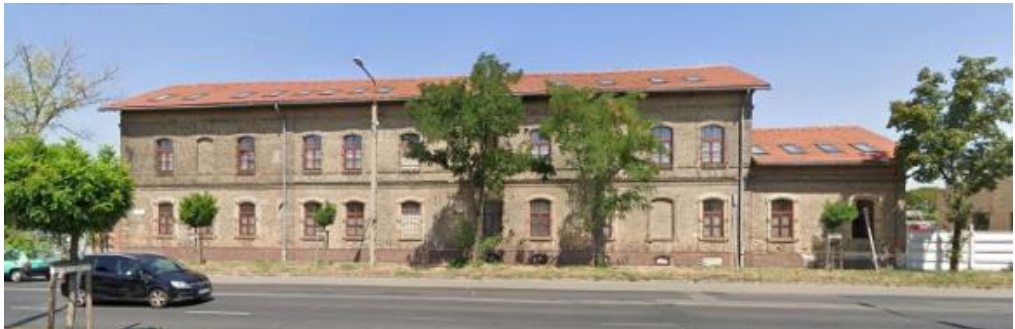
Fig. 1. The Hungarian demo building in original form.
