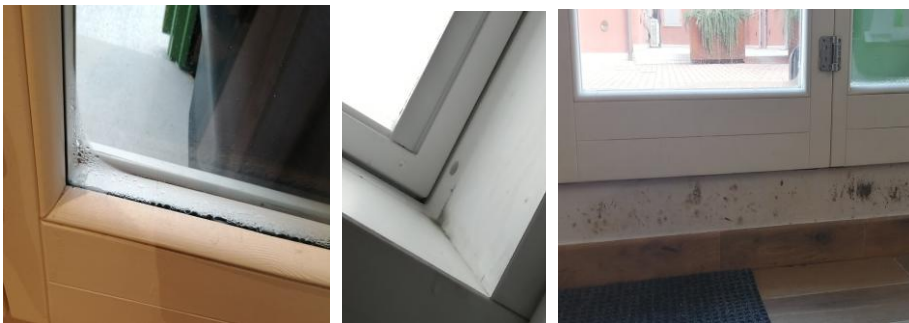
Fig. 4. Mold growth in an insulated single-family house renovated in 2025.
