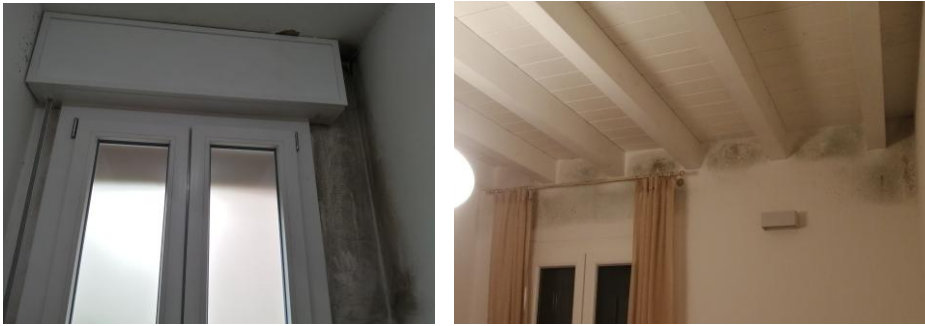
Fig. 3. Mold growth in a dwelling inside a multifamily building (on the left) and in a single-family house (on the right).
